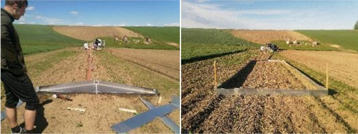
26.05.2021 Installation of the catchment area with dimensions: 3 x 10 m, using 1.5 mm thick and 2 m long steel plates.
