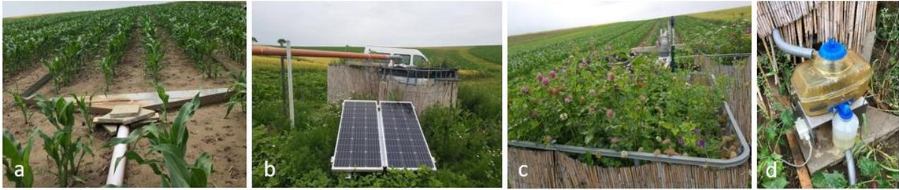
Figure 16. Catchment agricultural area, view of the agricultural runoff pipe that distributes the water on top of the three filter systems, PV island, vegetated filters, and tipping counter for effluent. 09.06.2022, Mistelbach, Austria.
