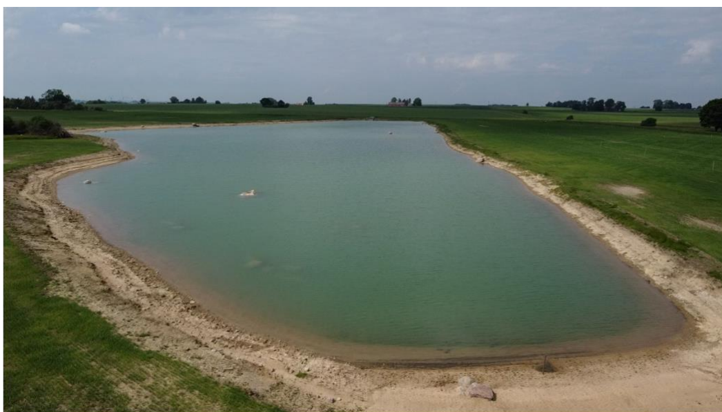
Figure 14 - Farm Constructed Wetland, Gårdstånga Nygård. The photo was taken soon after construction during the filling phase
